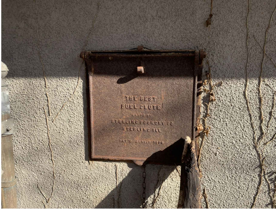
PHOTO #11 "FUEL CHUTE" LOCATED ON EXTERIOR LEFT SIDE OF GARAGE
