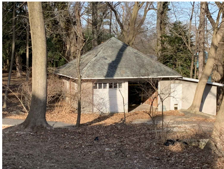
PHOTOGRAPH OF GARAGE TAKEN ON 2/15/23 FROM A SIMILAR LOCATION AS ABOVE PHOTOGRAPH FROM 1914
