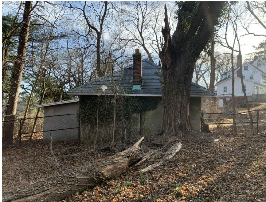
PHOTO #4 REAR ELEVATION
