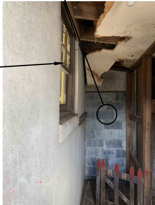
PHOTO #8 TYPICAL EXTERIOR WALL OF SHED ADDITION - CMU BLOCK
