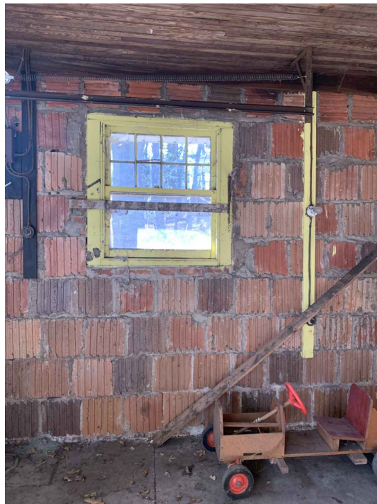
PHOTO #6 INTERIOR OF GARAGE
