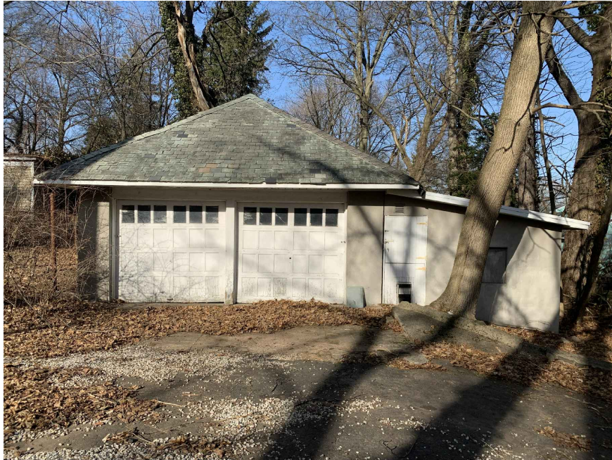
PHOTO #1 FRONT ELEVATION GARAGE CONSTRUCTED IN 1914 WITH SHED ADDITION ON THE RIGHT SIDE CONSTRUCTED AT A LATER DATE
