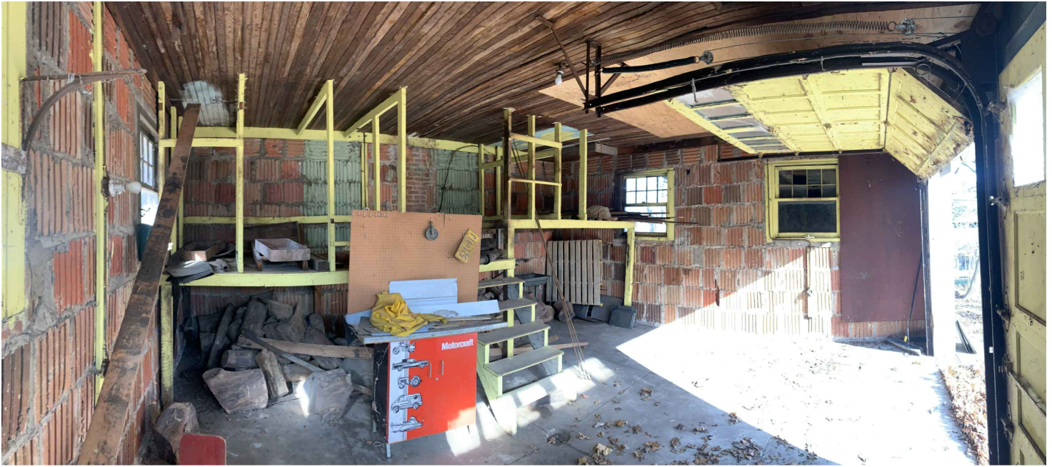
PHOTO #5 INTERIOR OF GARAGE
