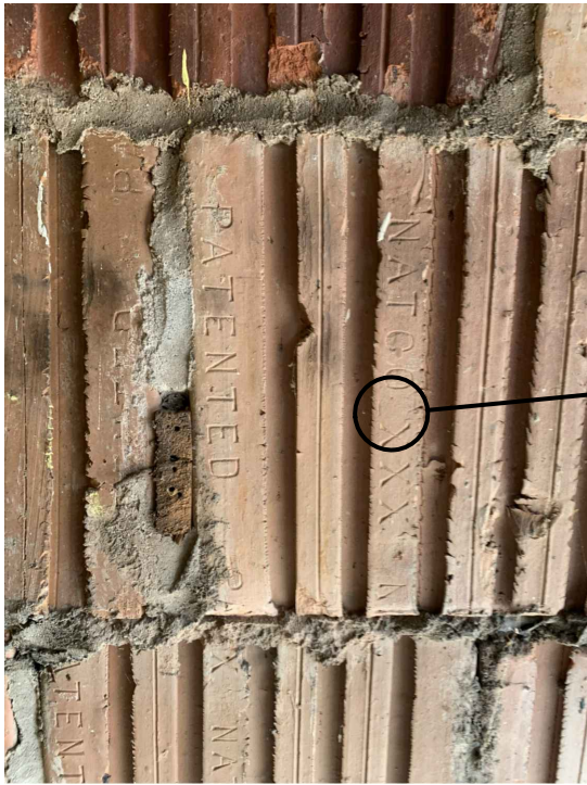
PHOTO #7 TYPICAL EXTERIOR WALL OF GARAGE STRUCTURAL TERRA COTTA
