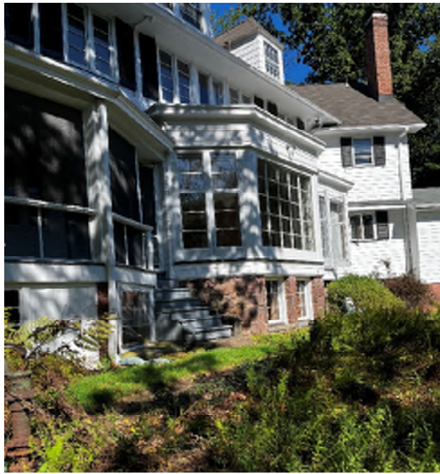
Photo#5 – Rear façade of 509 Park Street, Montclair New Jersey.
