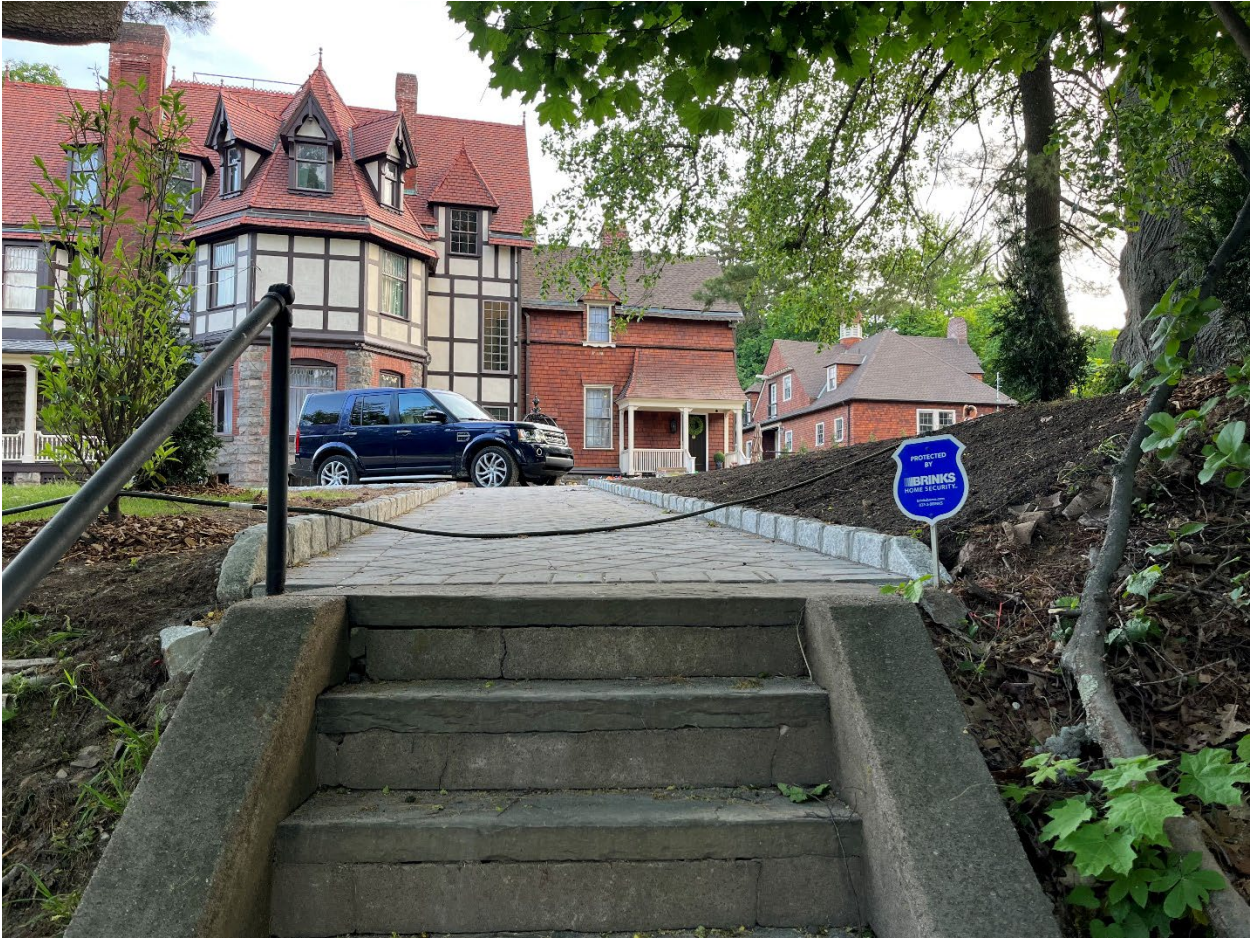
6) Images of Belgian block curbing at sidewalk from Claremont Ave and at parking area on north side of house
