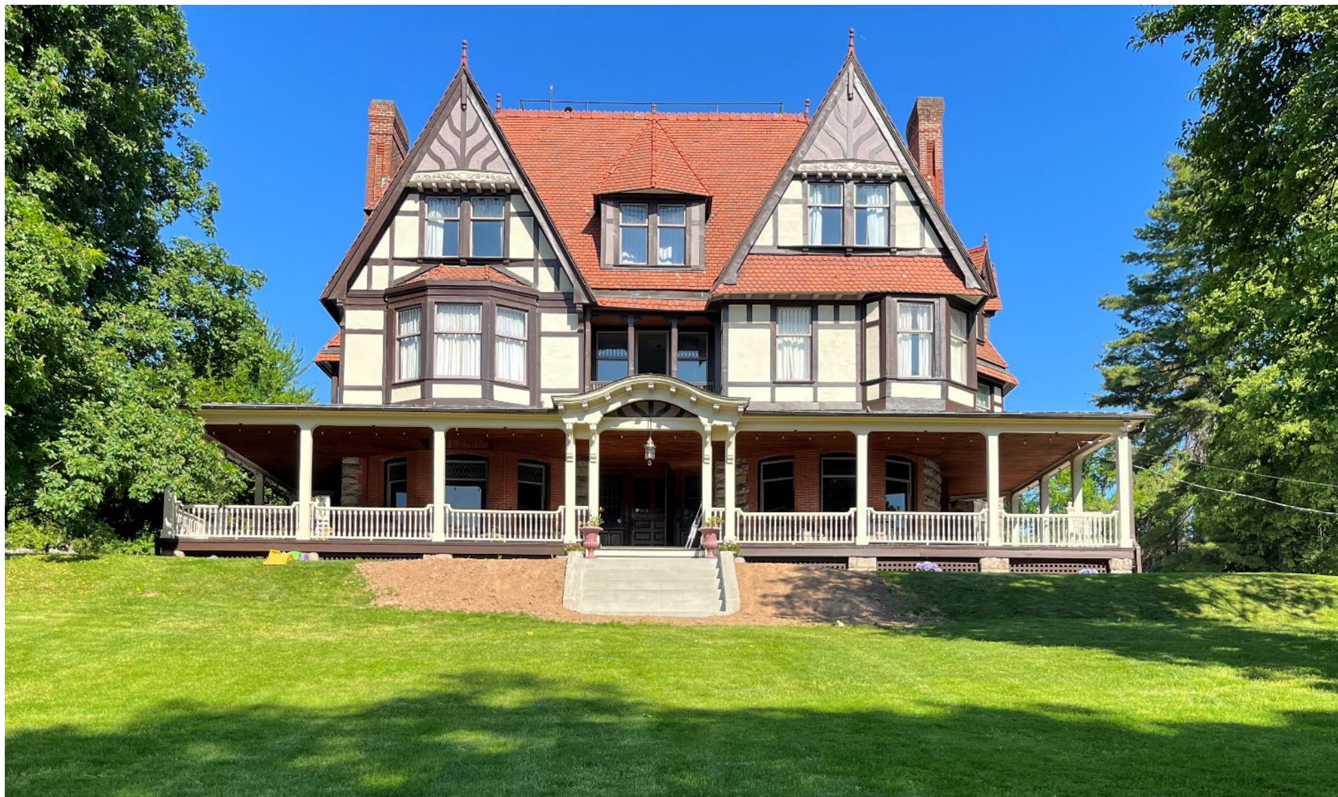
1) Image of concrete stair
