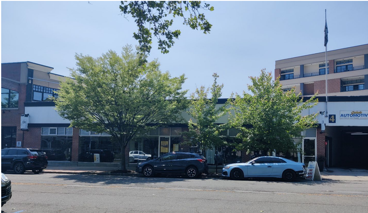
Figure 3: Gallery use in building at 4 Lackawanna Plaza.
