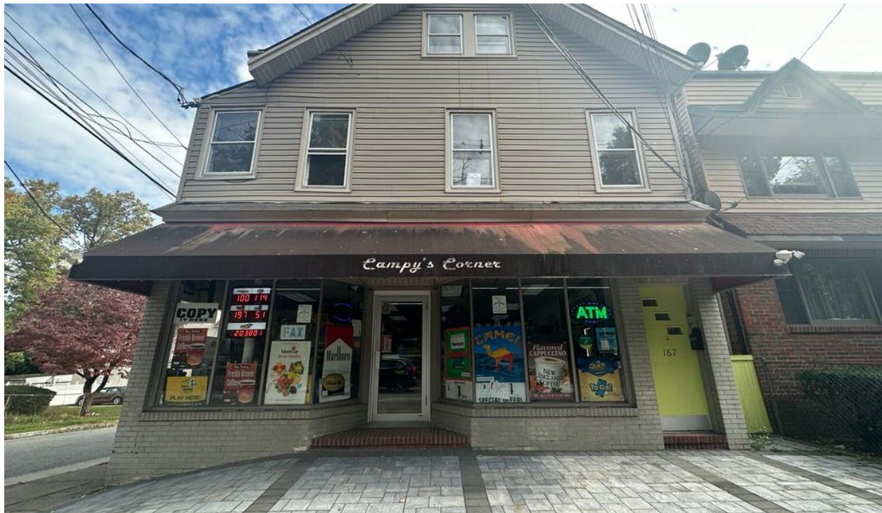
Figure 3: Mixed-Use property at 167 Harrison Avenue.
