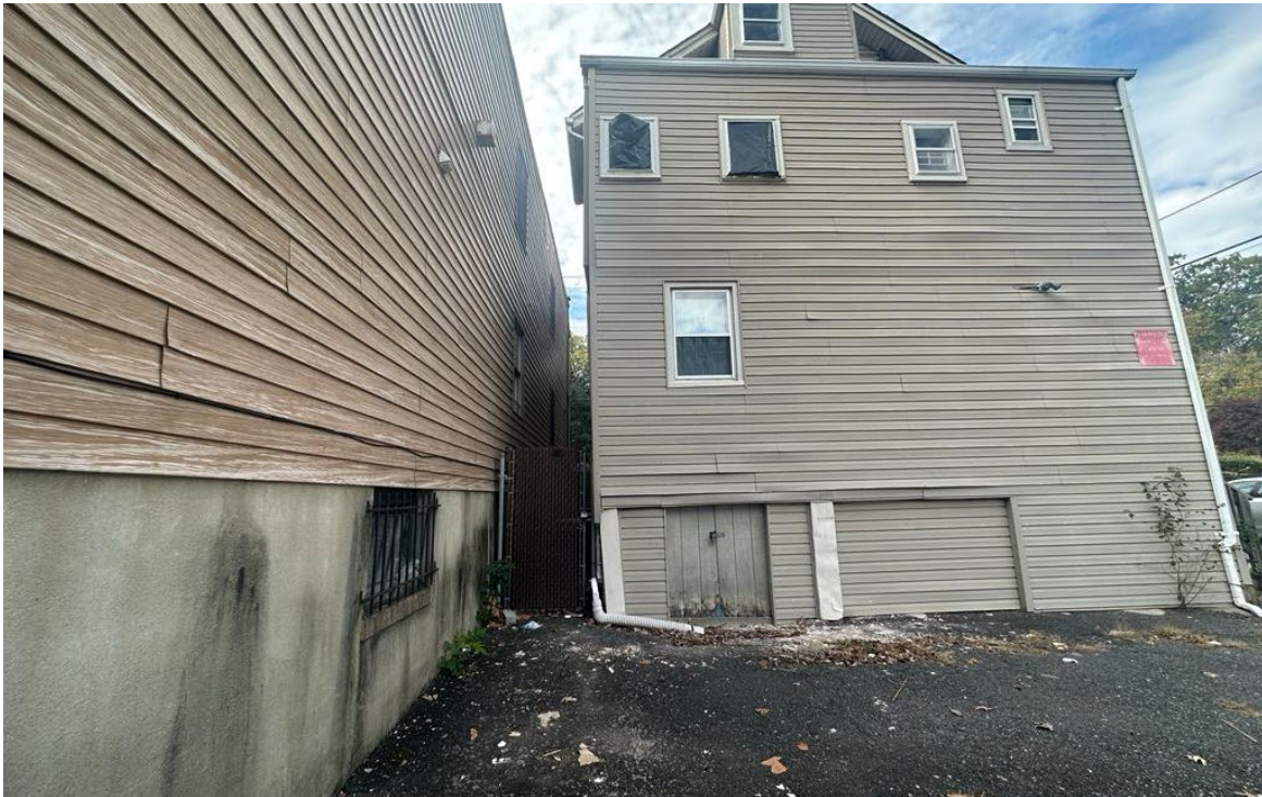
Figure 7: Parking side of the property with presumably storage and back door.
