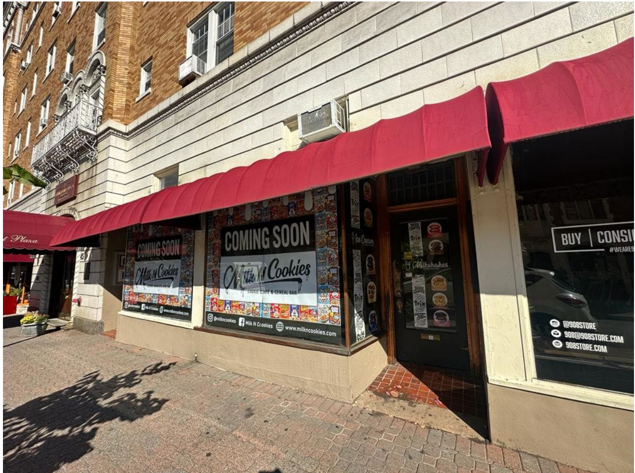
Figure 4: Commercial Building Storefront showing the door to be removed.
