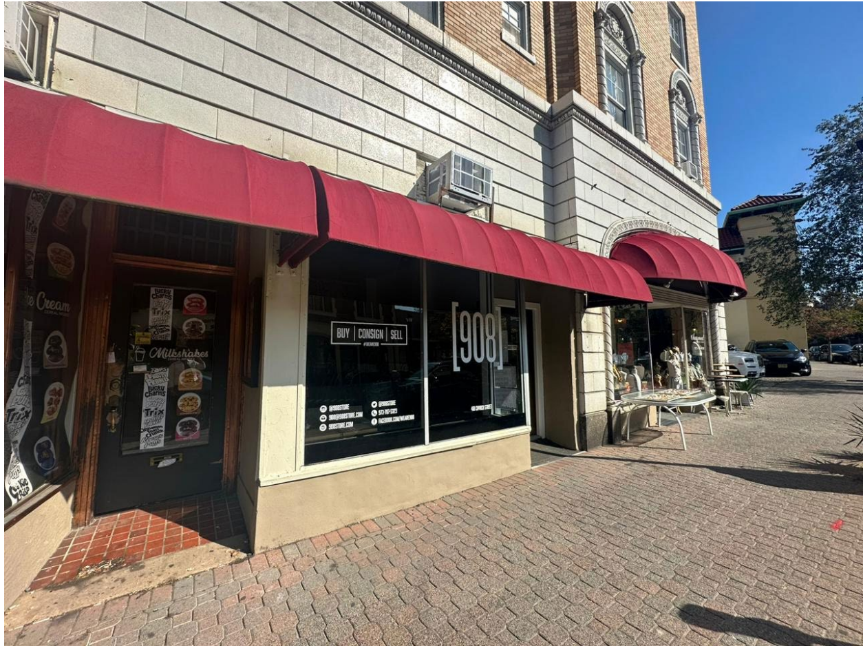
Figure 6: Signage on the shop beside 43 Church Street property.
