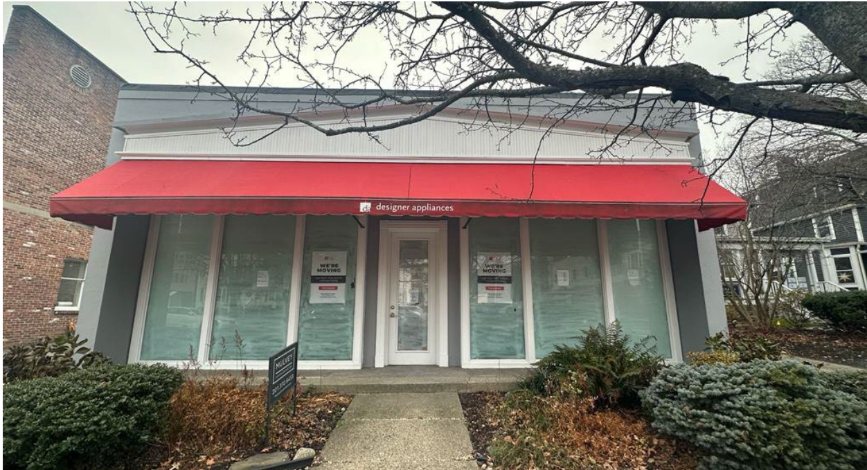
Figure 4: Front view of the subject property. Picture taken by staff, Dec 2023.
