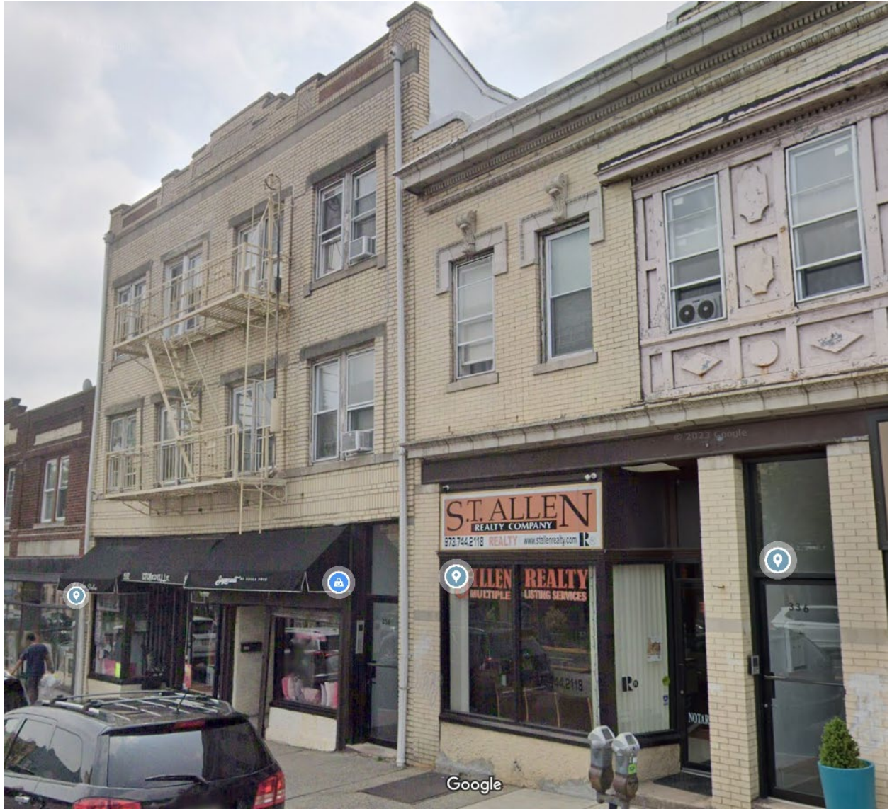
Figure 5: Property Storefront showing the front facade. Easterly Building (Google Images, June 2023)
