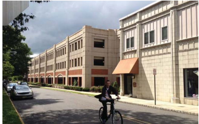
3.13-1: As a visible, free-standing structure, the Crescent Deck is widely appreciated in Montclair for its appearance and generous interior. It blends into its context by picking up on architectural cues from commercial and residential neighbors.
