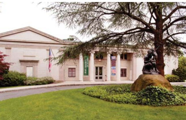
2.2-5: Sited prominently at the western "gateway" into Monclair along Bloomfield Avenue, the Montclair Art Museum's 1914 Neoclassical design serves as an example of the high standards the Township seeks in its built environment.
