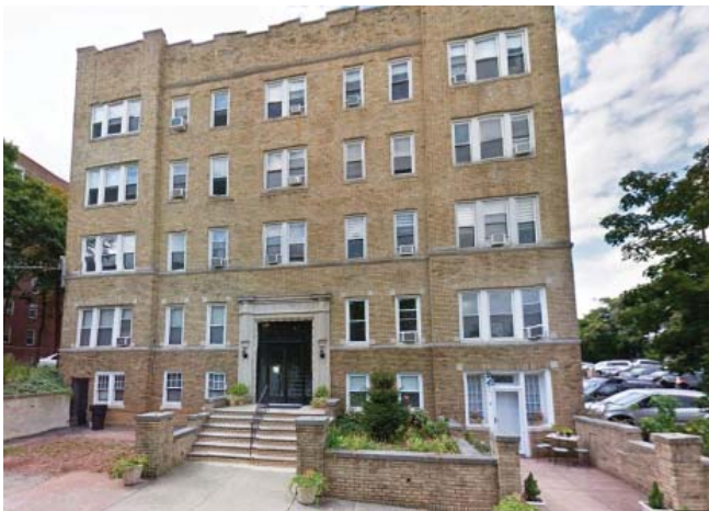
2.5.2-3: Multi-family apartment buildings along Seymour Street display what a bottom-middle-top strategy can look like when not employed by a mixed use building, as typically seen along Bloomfield Avenue.
