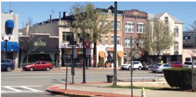
2.6-2: 381, 379, and 375-377 Bloomfield Avenue do not share the same size or awning detailing as their immediate neighbors, but utilize bottom-middle-top strategies seen elsewhere along Bloomfield Avenue.
