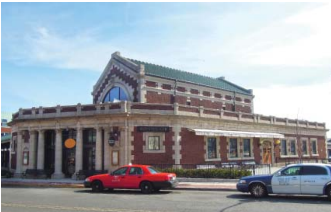
2.2-4: Although no longer serving its original function, the 1913 Beaux-Arts Lackawanna Train Station's high ceilings and arched, thermal windows create a dramatic interior space well-benefiting its bar and restaurant tenant.
