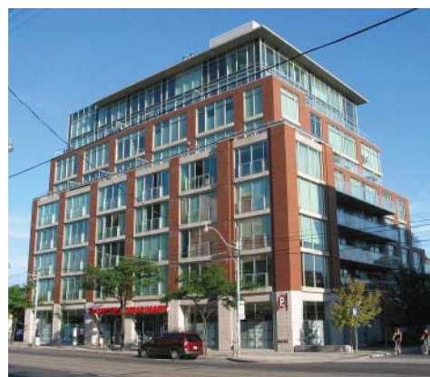
1.5-6: Discouraged: Uniform stepbacks on all sides of a building threaten to create a pyramid effect, highlighting overall mass rather than minimizing it. Where upper stories of a new midrise building will be visible from several directions, this must be avoided.
