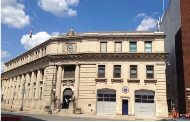
2.2-3: The 1913 former Municipal Hall, now Police Headquarters, at the corner of Valley Road and Bloomfield Avenue, handsomely combines Renaissance Revival proportions with Beaux-Arts detailing.
