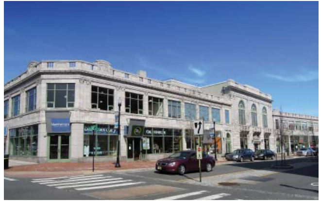
2.2-6: The 1926 Wedgewood Building's long, highly articulated Neoclassical commercial façade gracefully ties Church Street to Bloomfield Avenue along South Park Street. Its steady rhythm of decorative bays and storefronts sustains the walkable street.
