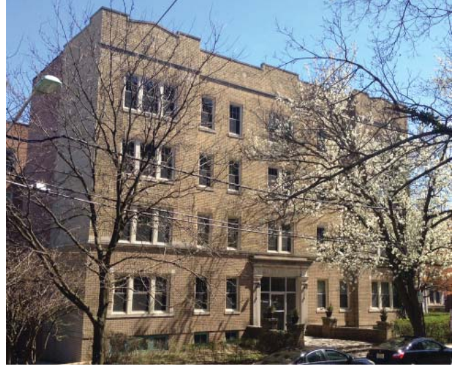
2.5.2-4: Shallow massing projections divide the building into vertical bays, breaking down the scale of the four-story structure. Stone framing the central entrance matches a stringcourse and the window sills, unifying the composition.
