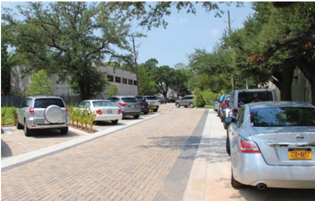
3.13-9: In this curbsless parking area, sidewalk and street are one. Changes in paving material, texture, scale and color serve to designate different zones of use. In this paved landscape, pedestrian and drivers have a heightened awareness of each other.
