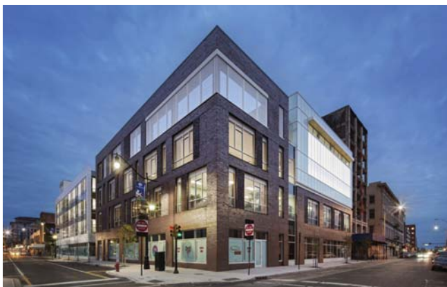
3.4-09: Historical material and style, such as brick and industrial openings, can be combined with new materials and expanded glazing to create a building suited for modern functions without seeming out of place in a walkable town center.
