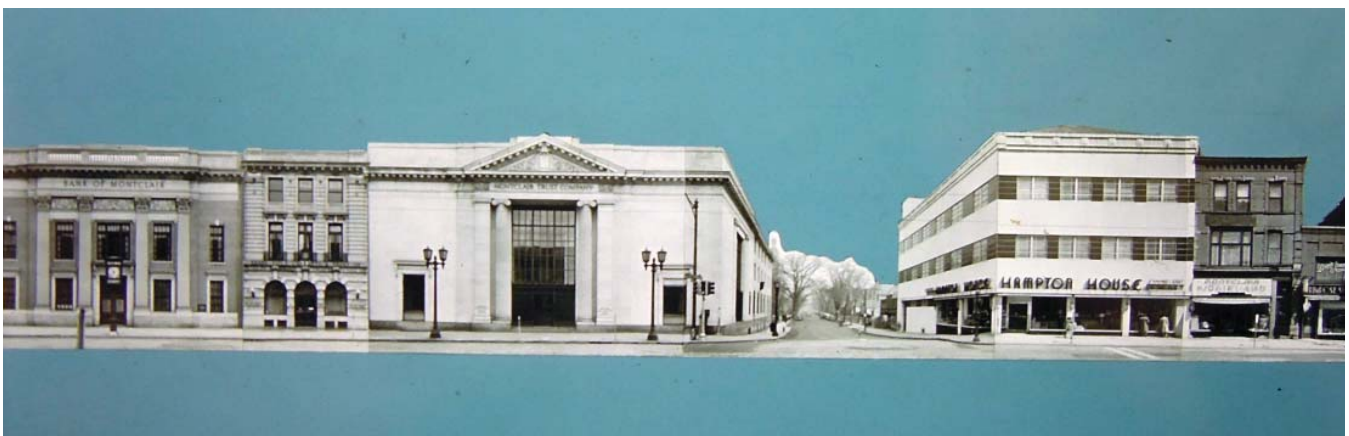
2.2-1 and 2.2-2: As seen c.1946, the north side of Bloomfield Avenue, between North Fullerton Avenue and Park Street, displays an eclectic mix of architectural styles created over 50 years of spirited Town Center investment and development.
