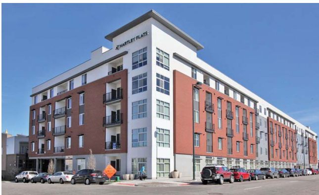
1.3-2: Discouraged: Brick is often employed across the country to imitate existing traditional architecture. However, if lacking in detail and paired with other plain surfaces, brick alone cannot provide the depth and character of our nation’s better buildings.
