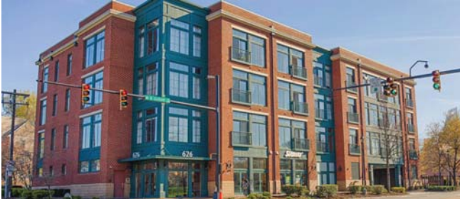
3.7-1: A recessed vertical bay element, similar in width to the building's standard bay, unobtrusively highlights the corner.
