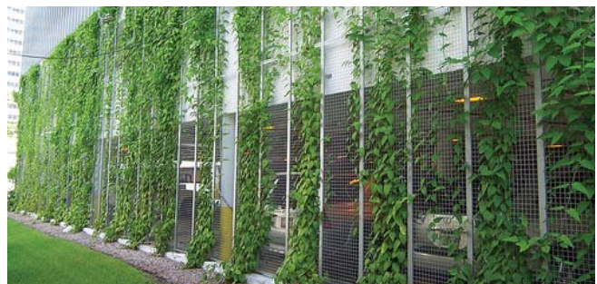
3.13-3: A “green” screen applied to a parking structure both shades the interior and softens the spaces around the deck.
