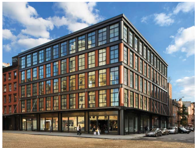
3.4-05: Holding the corner of a block in Tribeca, this transitional design borrows the proportions and materials of nearby historic cast iron loft buildings. In the middle floors, brick piers substitute for cast iron, a nod to adjacent masonry buildings.
