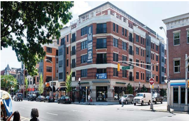
1.5-3: Encouraged: Stepbacks must be combined with clear form or detail to work effectively. The above example uses punched window openings, a stringcourse at its second floor, and a cornice at the top of the fifth floor to relate to an older building (at right).
