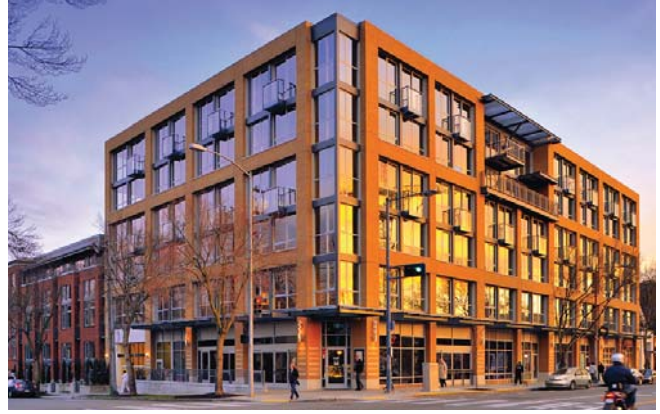
3.4-07: Borrowing from historic factory design and the modern office building, this Interpretive Modern building uses traditional materials and a multi-layered facade to fit within its neighborhood, despite being larger and not relying on setbacks.
