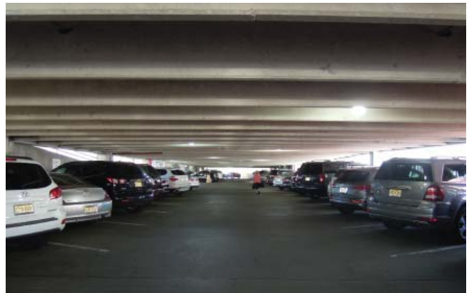
2.8-3: Minimal floor to floor heights within the North Fullerton Deck create dim spaces that don't feel safe.
