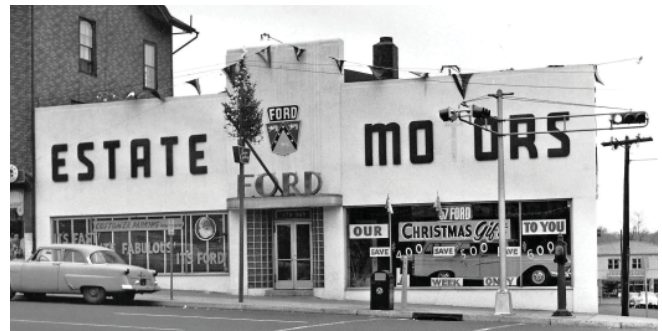
2.6-4: 369 Bloomfield Avenue previously embodied the Art Moderne aesthetic that briefly bloomed in Montclair, along with the Hampton House. The wide storefronts, glass block and bold signage are classic features of the style.
