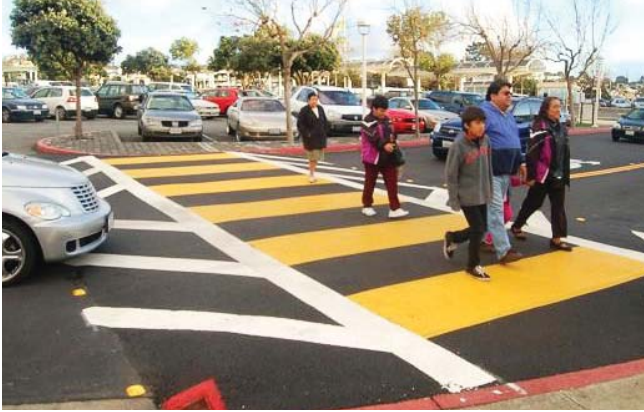
3.13-8: This wide speed bump doubles as a pedestrian path cutting through a parking area. Shallow asphalt ramps, diagonal striping and broad colorful bands highlight the walking zone, ensuring that drivers are both physically and visually aware of the path.
