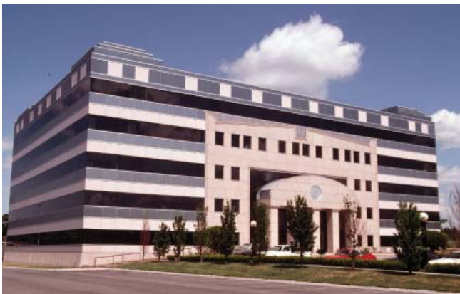
1.6-1: Discouraged: Requiring buildings to imitate or integrate historical styles and elements can lead to designs that seem like cheap parody.
