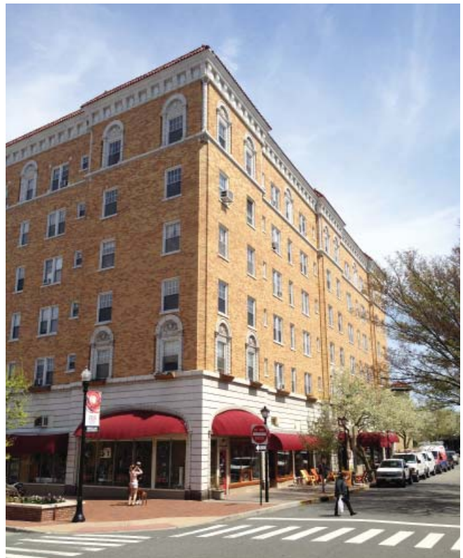
2.5.2-1: At six stories tall, the Claridge Apartments is one of the tallest buildings in Montclair. However, material choices, window placement and detailing allow the building to fit within its context without a single stepback.
