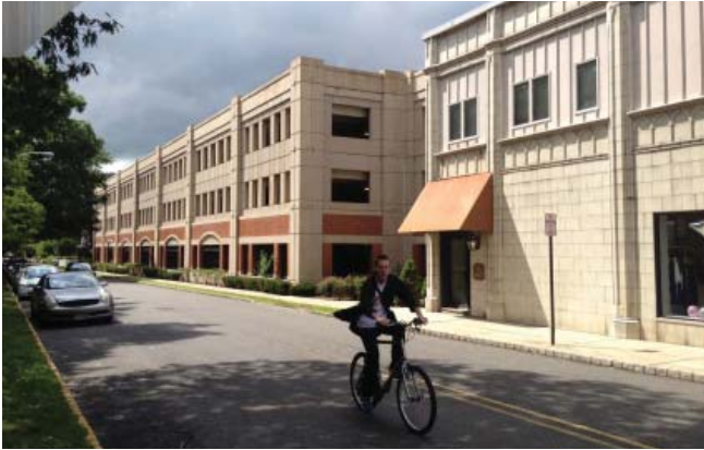
2.8-5: Along The Crescent, the Crescent Deck utilizes the architectural lessons from its commercial neighbors, extending the street-wall and emulating older architecture through modern precast concrete detailing.
