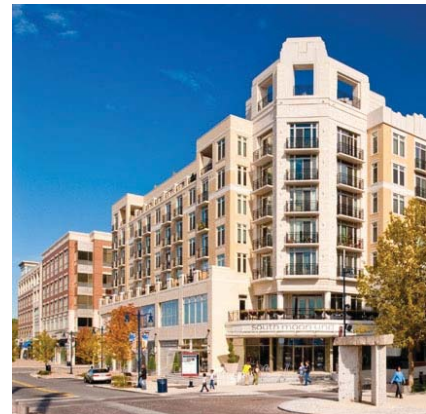
1.5-4: Encouraged: A prominent corner transition employs a deep entrance canopy and third-story stepbacks on the side to create a welcoming streetscape and an architectural rhythm easily legible to pedestrians.
