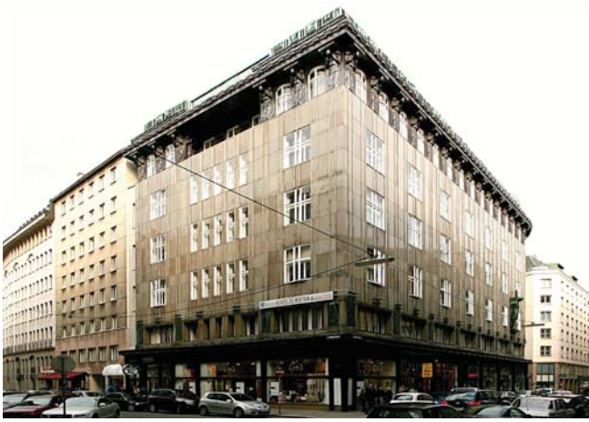
3.4-06: Interpretive Modern design knowledgeably reinvents historic design. This mixed-use structure shares the base-middle-top composition of its older neighbors but amplifies its storefront and cornice to capitalize on the corner location.
