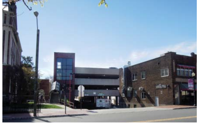
2.8-2: The North Fullerton Deck's deep setback leaves it hard to find and foreboding. The Deck's proximity to an adjacent building creates a curb cut too close to Bloomfield Avenue, resulting in a cramped approach and increased traffic.
