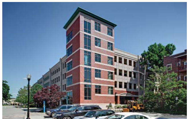
2.8-4: The Crescent Deck picks up on architectural cues, including massing, detailing, and material use, from neighboring traditional multi-family housing. The deck's location presents a more natural approach, away from heavily used thoroughfares.
