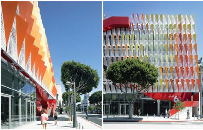
3.13-5: A repetitive system of three-dimensional elements is a powerful way to screen a parking deck. Depending upon the viewing angle and the use of color and form, the screen will change appearance from different vantage points.
