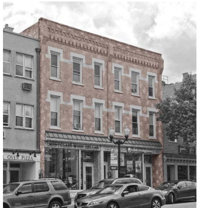
2.4.2-3: Buildings do not require expensive carved stone or molded masonry to create a contextual facade. Brick pilasters, draped lintels and a corbeled brick cornice at 440-444 Bloomfield Avenue make for a handsome, harmonizing building.
